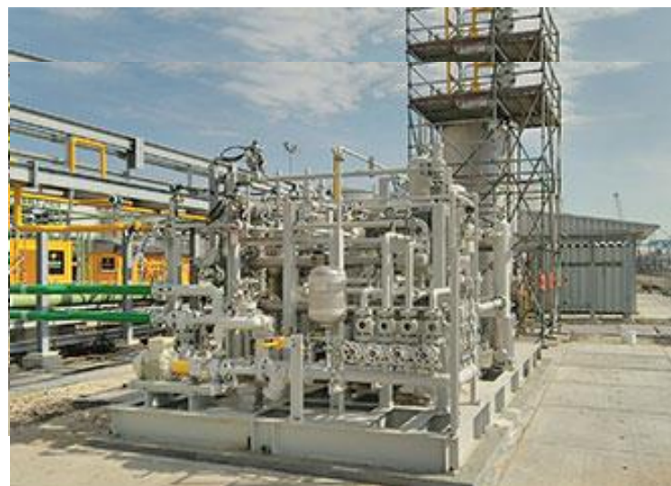
“MultiPLHY”, World’s largest High-Temperature Electrolyzer
